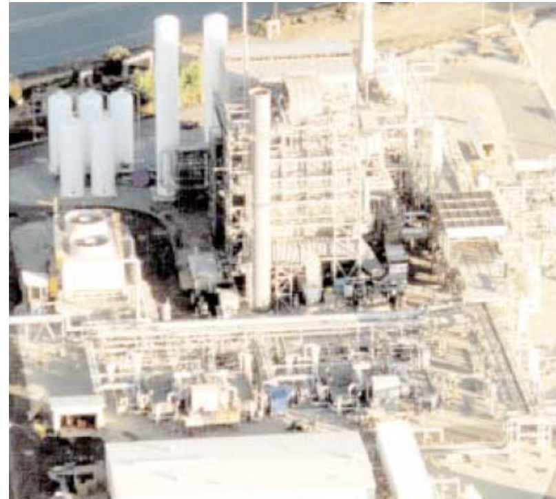
Air Products 96 MMSCFD SMR in Carson, CA is connected to a pipeline with another Air Products SMR, allowing refineries to meet environmental regulations and enjoy benchmark reliability.
